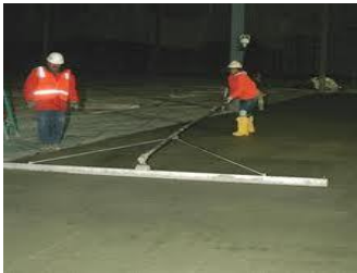
Figure 2 Smooth Steel Floated Floor Surface
