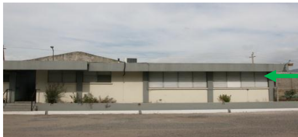
Figure 3 Windows being a third (1/3) of the Wall Space to Facilitate Air Flow
